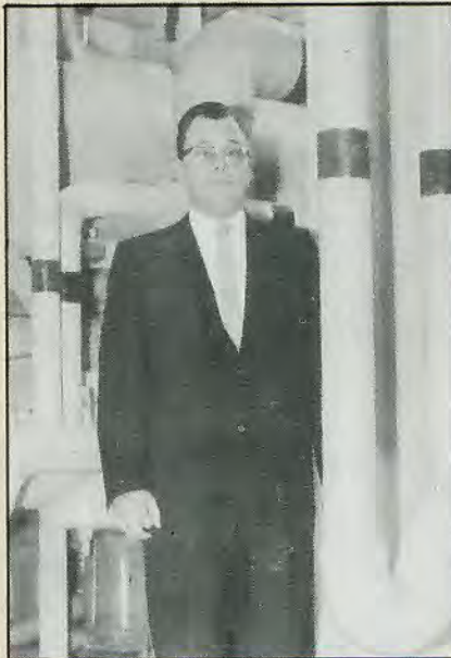
Jack Thompson inside refrigeration piping/machinery room of Arkansas Power & Light Company in Little Rock, Ark. The 1958 project utilized a unique two-stage heat pump system.
