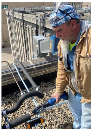
Starco installer Dave Hirby uses a NIBCO PCR-20M Press System® battery-operated, mini pressing tool to install PressACR® fittings for joining copper tube systems in air conditioning and refrigeration applications.
