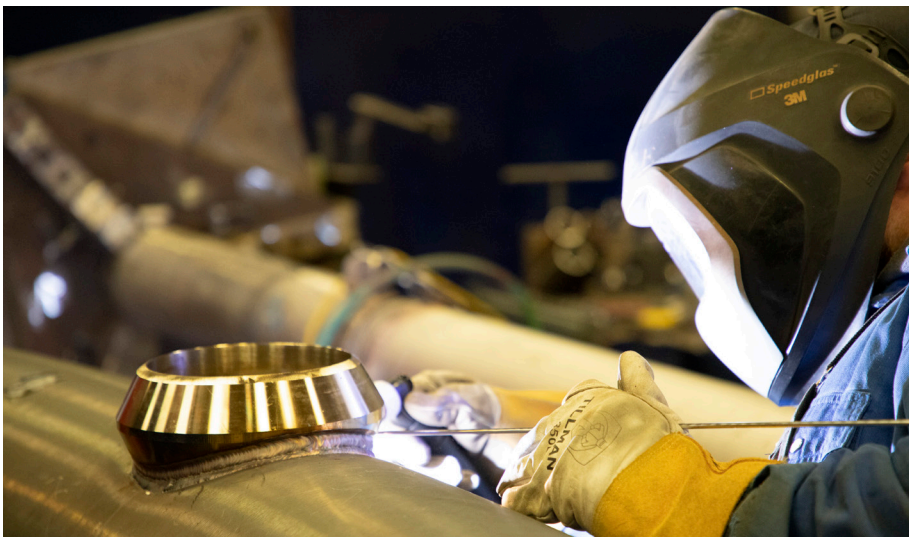
Harris found that the quality of cuts made by the Watts Specialties pipe cutter dramatically reduced the work needed for pipe fitup in preparation for welding.
