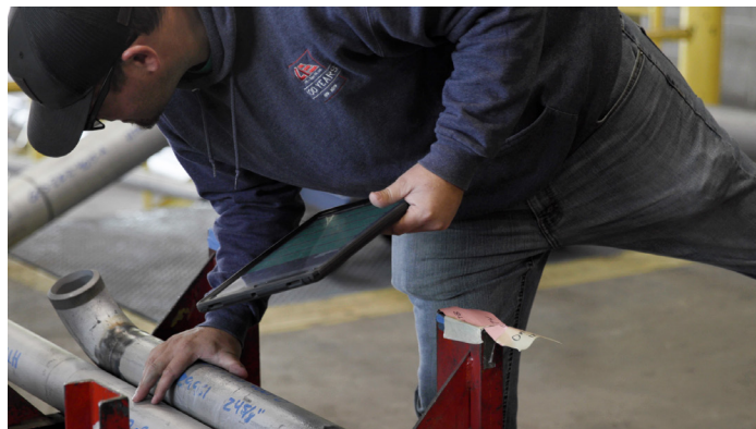
Shane Shook, CWI, Egan superintendent, examines the quality of a pipe weld. By using MSUITE, Egan has improved quality control and tracking, which is crucial for large industrial clients.
