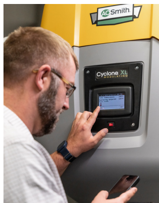
Hampton Inn General Manager Sammy Naquin uses A. O. Smith’s iCOMM Connectivity Platform to adjust the Cyclone XL water heater’s settings; the application also allows him to monitor and revise settings remotely.
