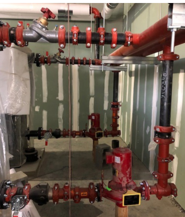
Thanks to Victaulic’s VDC team, Maxair was able to optimize the mechanical room layout for the School of Medicine, so each component is easy to access and can be disassembled without welding or flanging, simplifying maintenance and service.
