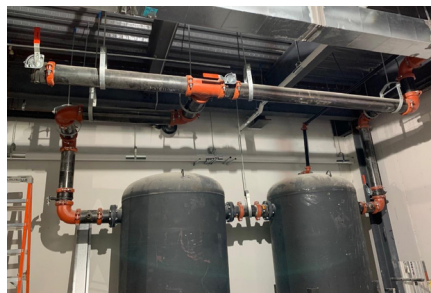
Maxair Mechanical used Victaulic grooved couplings, fittings, and valves to tie in two boilers inside the first-level mechanical room at Mercer University's School of Medicine, saving time compared with welded solutions.
