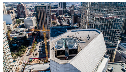
Using two Marley NC Cooling Towers, Graco Mechanical met the Lyric Tower's need for new, efficient cooling towers that could be installed inside the existing mechanical pit without altering too much of the existing piping arrangement and structural steel.
