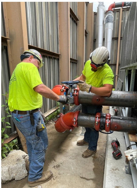
General Piping’s Jason Miller (left) and Newt Briar installed NIBCO’s #GD4765-5 grooved butterfly valve on the exterior chilled water piping that feeds the high school’s new air-cooled chillers. The ease of installing the NIBCO products helped General Piping stay within the narrow window for completing the cooling system.
