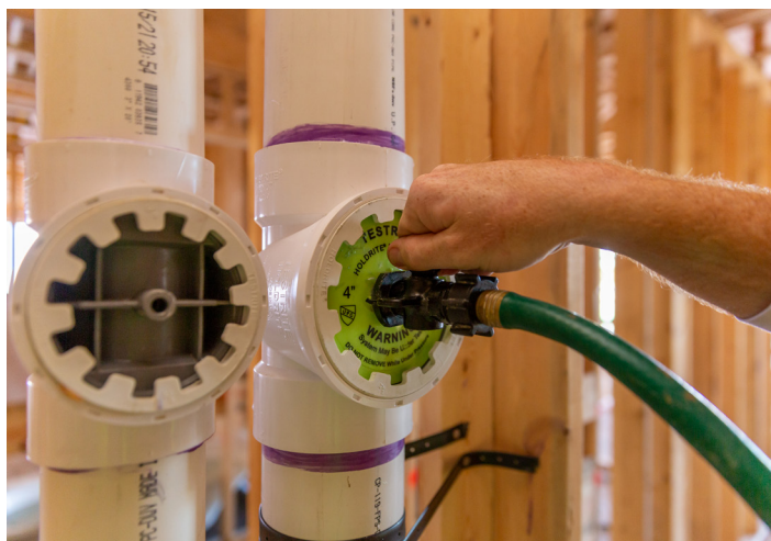
Modern methods for DWV testing for new pipe installations, such as HoldRite's TestRite system from RWC, are faster, easier, and safer than the traditional approach using inflatable test balls.
