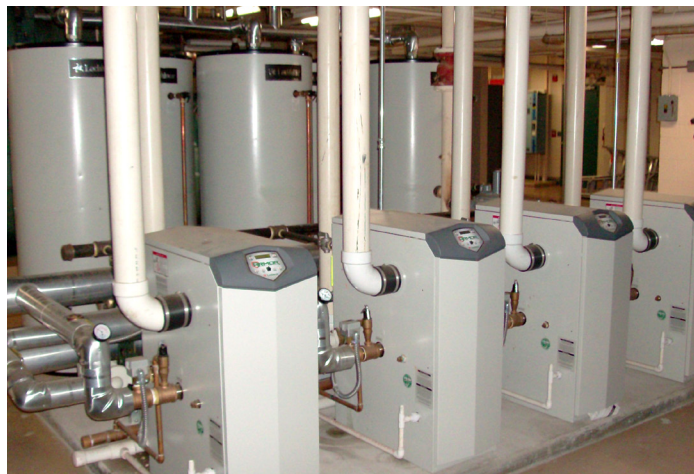
Nashville Machine Company had to cut Vanderbilt University's old water heater and storage tank into pieces to get it out of the mechanical room. They replaced it with four Lochinvar ARMOR water heaters and five storage tanks small enough to fit through the mechanical room doors. The flexibility of ARMOR's venting options allowed for a smooth, successful installation.
