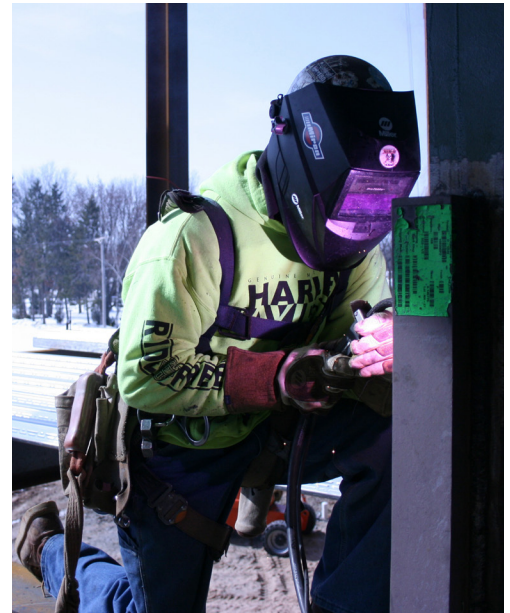
Converting to wire welding processes is one change that contractors can make to improve productivity and efficiency.
