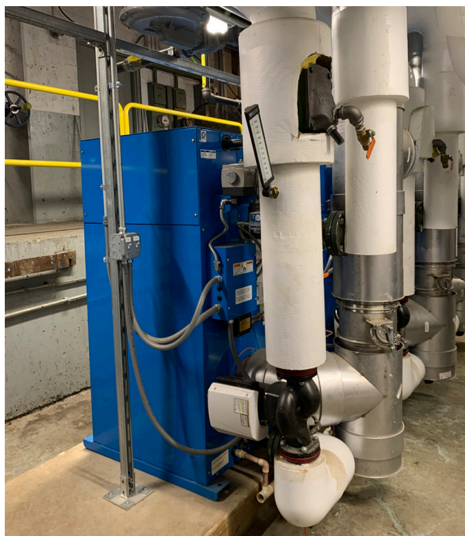
AMS solved a Chicago condominium's recurring pump failures with Metraflex's LPD Mag Retrofit Kits—an easy-to-install, low-cost fix that keeps metal debris out of the pump motors.
