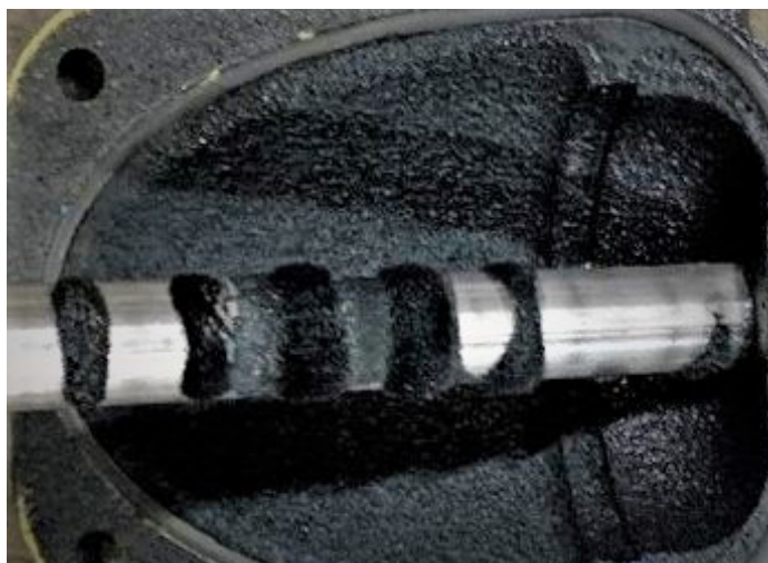
AMS retrofitted existing Y-strainers with Metraflex’s LPD Mag Y-strainer, which has a neodymium magnet that attracts metal particulates before they reach the pumps—an easy solution to the persistent pump failure problem. This photo shows the cover plate before blow down.
