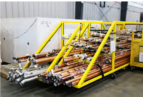
Prefabricating with Viega ProPress meant that the Olson crew spent less time working at altitude to complete the Pikes Peak Summit Complex, where the air was thin and the weather potentially dangerous.
