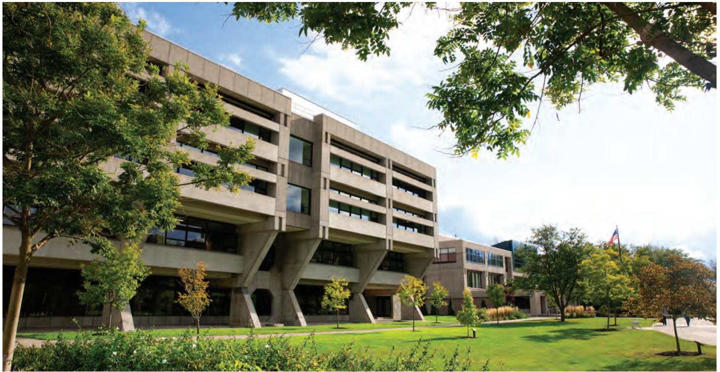
EMCOR Services-Betlem helped Finger Lakes Community College move its ambitious sustainability plans forward by specifying a Lochinvar cogeneration system for hot water and heating, earning the college a $17,000 design/build incentive from the state utility and projected electricity savings of more than $11,000 per year.
