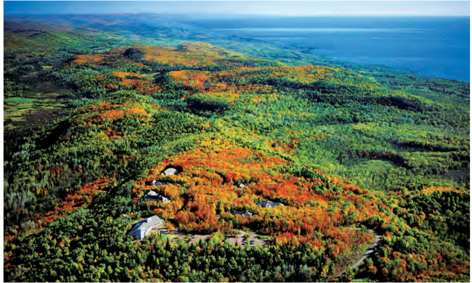
McKinstry specified Uponor's Ecoflex preinsulated PEX piping to resolve persistent heat retention problems at Wolf Ridge Environmental Learning Center in Finland, MN, where winter temperatures can fall well below zero for months and seasonal snowfall accumulations can total more than 100".
