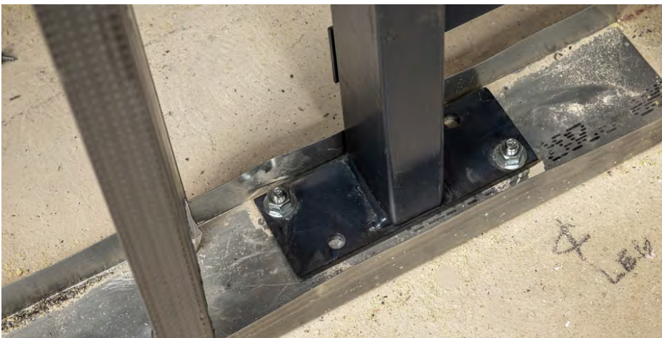
J.M. Brennan saved time during installation with the Z1231EZ Universal Lavatory Carrier, which uses two foot-anchors per upright instead of four.
