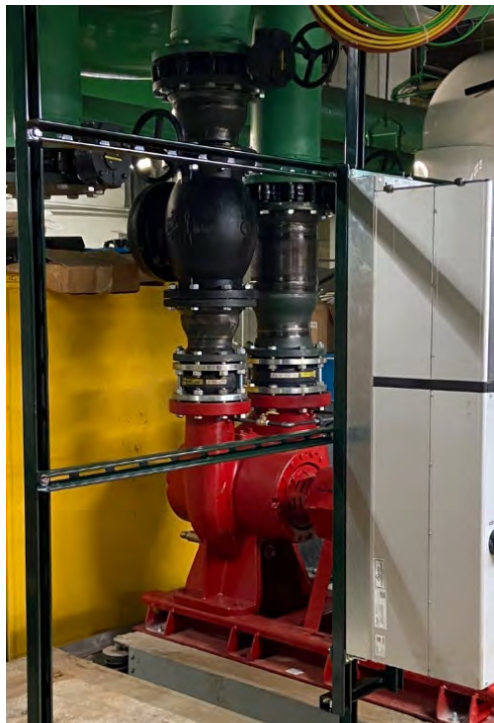
These examples all show check valves that are installed too close to the pumps. In all three, reducers were installed between the pump and the check valve, suggesting that the check valves were likely oversized for these pumps.
