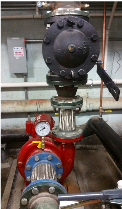
These examples all show check valves that are installed too close to the pumps. In all three, reducers were installed between the pump and the check valve, suggesting that the check valves were likely oversized for these pumps.
