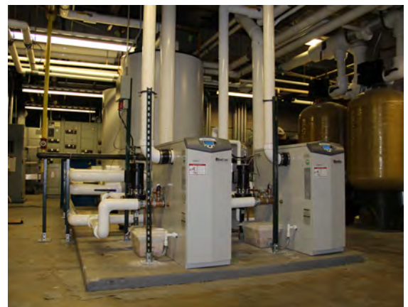
Left: Lexington Plumbing installed two new, efficient Lochinvar ARMOR water heaters to meet the high demands of the Wyandotte (Kansas) County Jail while keeping operating costs low.
