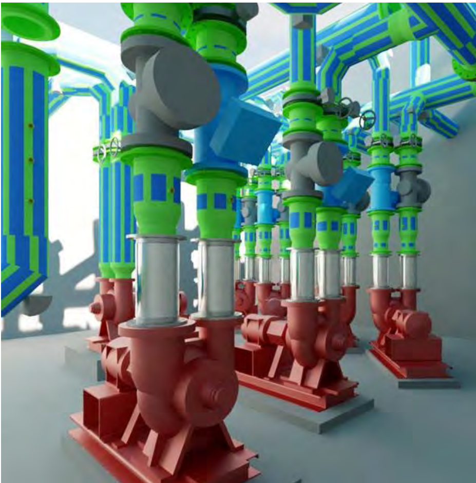
Using Ferguson's new VDC capacities helped MMC avoid potential problems at the planning stage of a large project, saving the contractor time and money.
