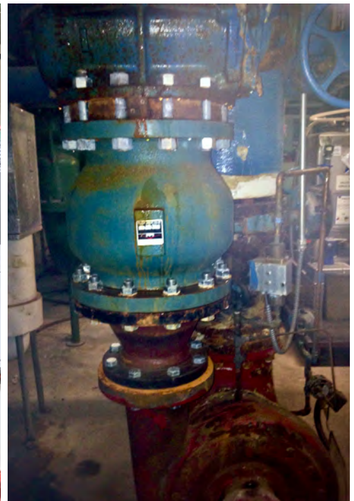
These examples all show check valves that are installed too close to the pumps. In all three, reducers were installed between the pump and the check valve, suggesting that the check valves were likely oversized for these pumps.
