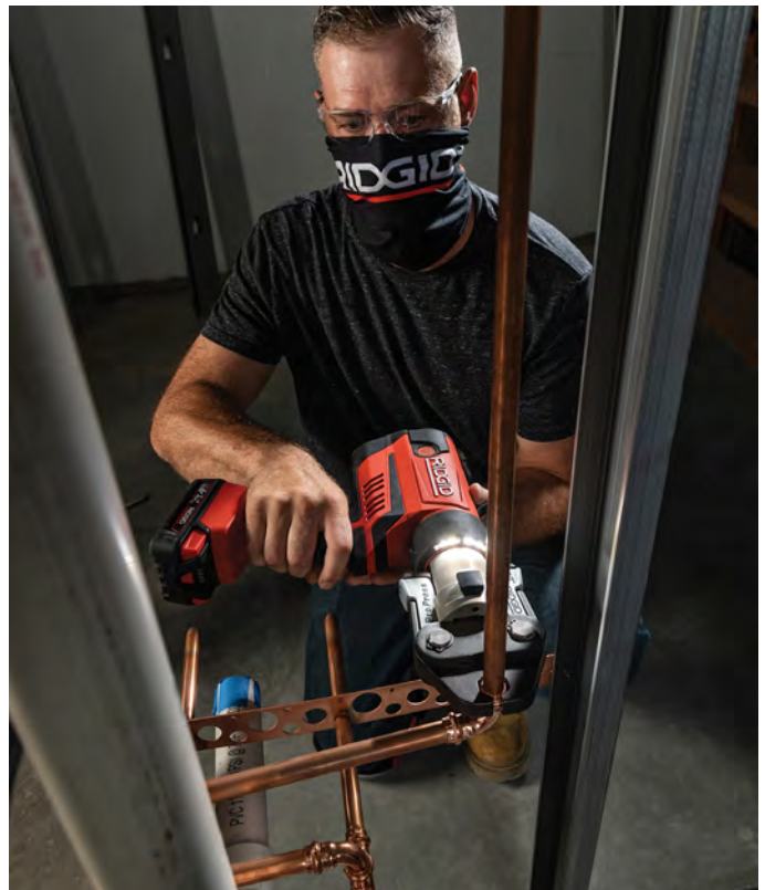
You can increase productivity by choosing tools that need little or no maintenance—such as the RIDGID RP 350 Press Tool, which has a brushless motor that eliminates the need for scheduled service.
