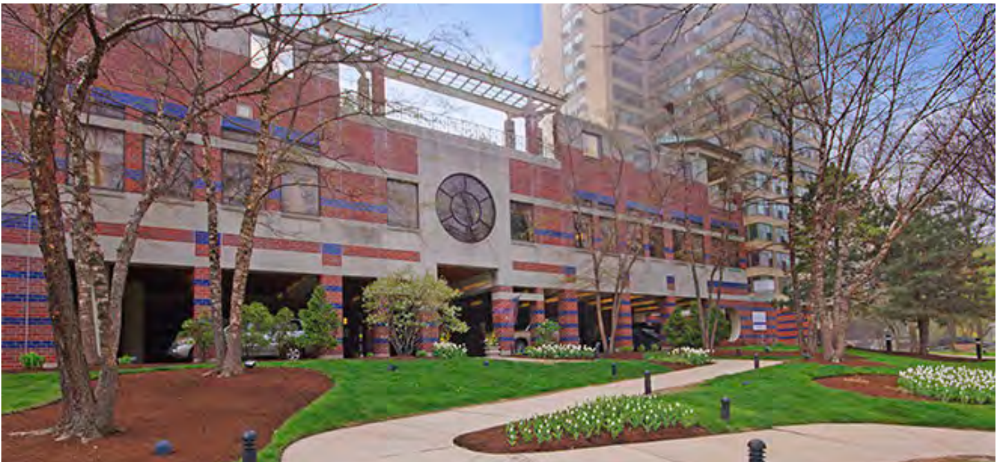
Through careful planning and coordination with the city, Daikin successfully installed a new chiller in the Brookdale Senior Living Center in Chicago with minimal disruption to the senior residents and their neighbors.
