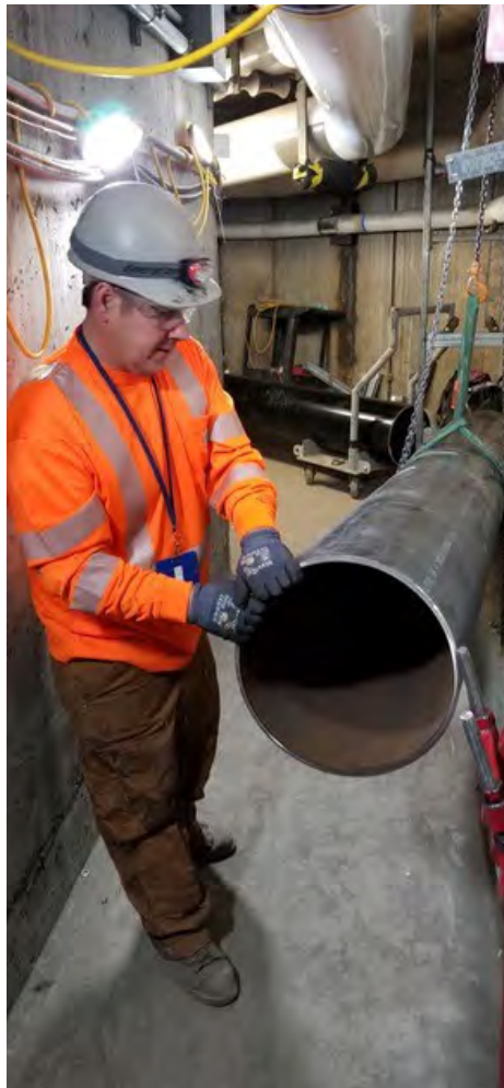
Left: Hermanson Company's staff paired a space-saving Miller Electric welder with a novel mechanism to rotate pipe in place, making welding easier in a confined space for Gary Lockram, UA Local 32, and coworkers, which increased productivity.
