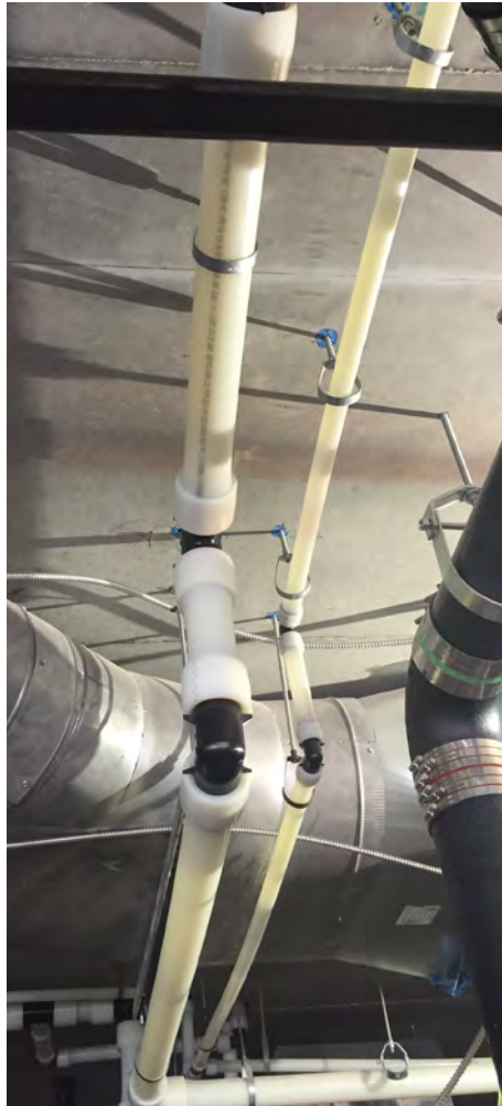
Left: By using Uponor PEX for a new high school’s plumbing, Letsos Company avoided the need for torches or glues, increasing the speed and safety of installation.
