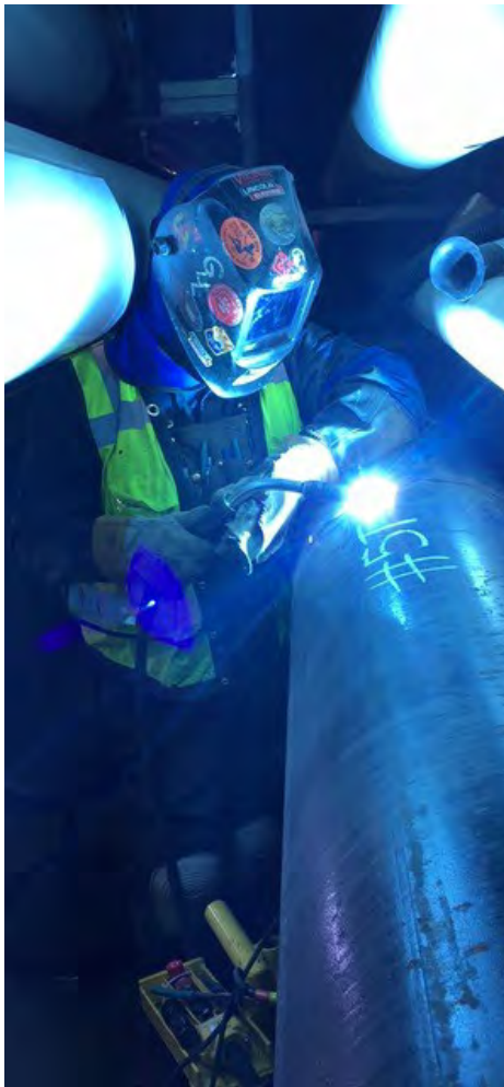
Left: Hermanson Company's staff paired a space-saving Miller Electric welder with a novel mechanism to rotate pipe in place, making welding easier in a confined space for Gary Lockram, UA Local 32, and coworkers, which increased productivity.
