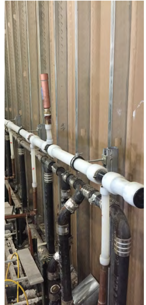
Left: By using Uponor PEX for a new high school’s plumbing, Letsos Company avoided the need for torches or glues, increasing the speed and safety of installation.
