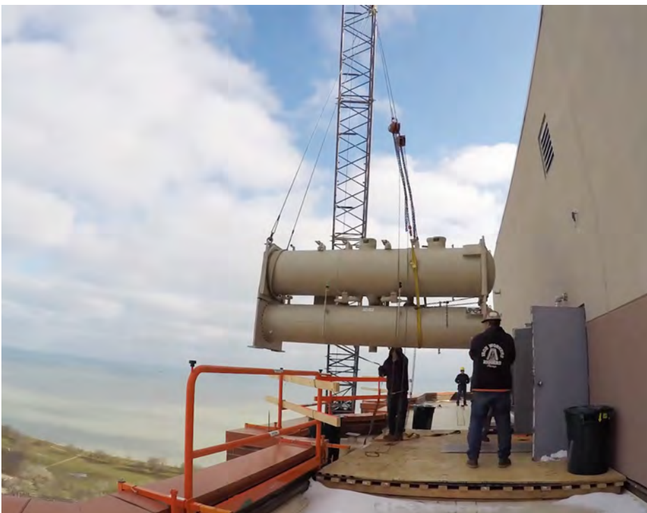
Bottom: Replacement of the Brookdale Senior Living Center’s 30-year-old chiller with a new Daikin Magnitude® magnetic bearing water-cooled chiller stayed on time and within budget thanks to advance planning and Daikin’s expertise.
