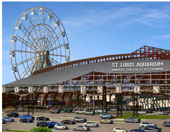
St. Louis’ new aquarium opened on time thanks to a solid collaboration among Anvil International, Rock Hill Mechanical, and National Sales Company. Anvil’s Gruvlok products helped speed up installation in the mechanical room.
