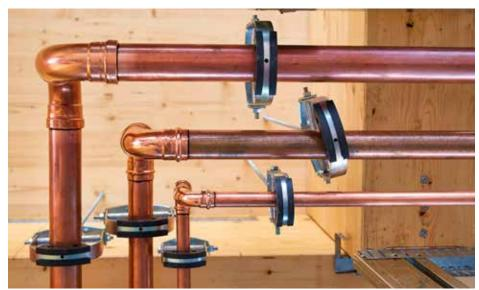
Viega's two new buildings use ProPress fittings behind the walls to provide potable water because, as Braconier President Tom Stone said, soldered joints might leak, but ProPress joints do not.
