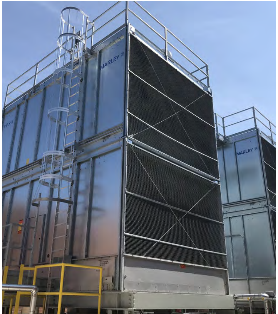
IFS replaced 40-year-old wooden towers at a St. Louis, MO, government building with a two-cell Marley NC 8414 steel crossflow cooling tower, factory-assembled by SPX Cooling Technologies Inc.—while keeping the chiller system operational throughout to avoid disrupting essential county government services.
