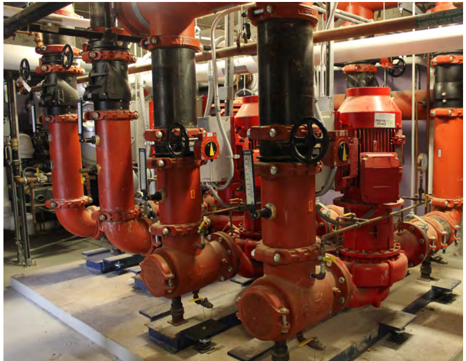
Victaulic products, including these vibration isolation pump drops, and close collaboration with Victaulic's design team helped Poole and Kent finish the mechanical room installation for the new Baltimore high-rise apartment complex in only 50 days, 15 days ahead of schedule.
