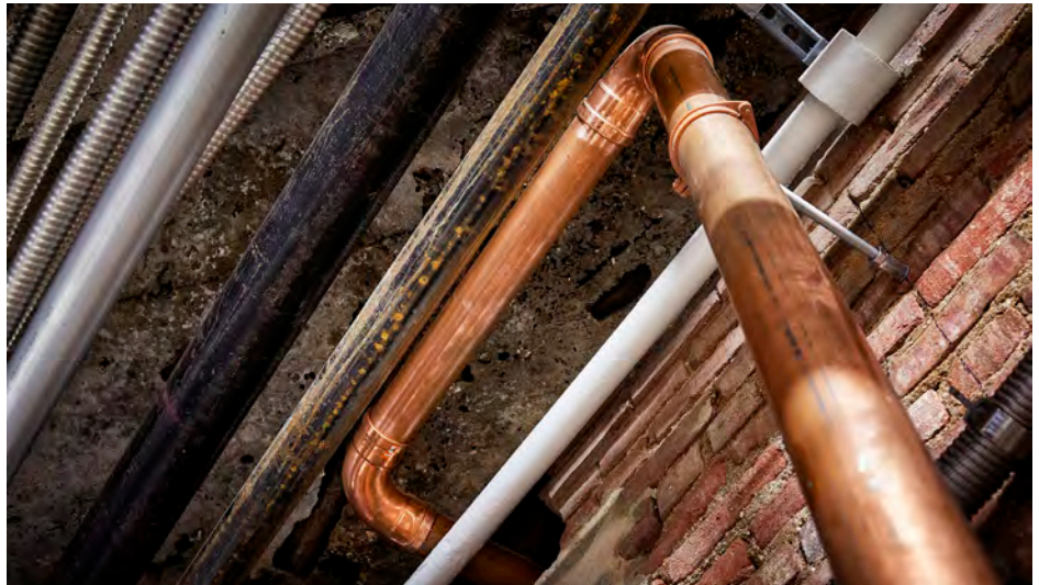
Devine Brothers said using Viega ProPress to install about 15,000' of copper pipe for the massive replumbing of the Philadelphia Metropolitan Opera House saved time and money.
