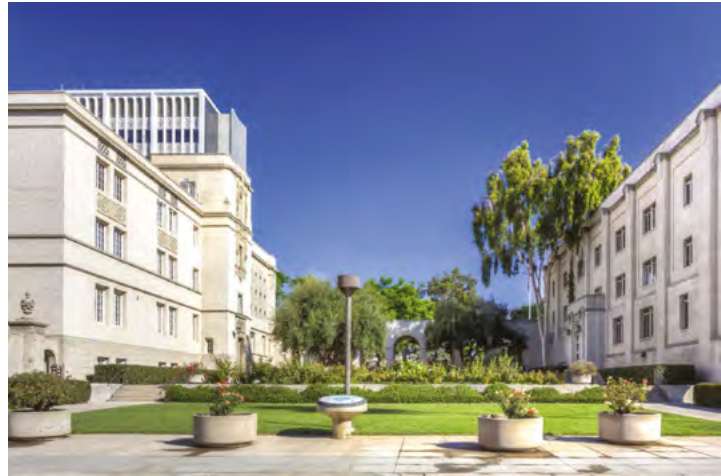
Since Muir-Chase Plumbing installed Zurn Retrofit Pint urinal systems in every bathroom across campus, Caltech, the world-renowned science and engineering institute in Pasadena, is saving 6,056,130 gallons of water and $42,393 per year.
