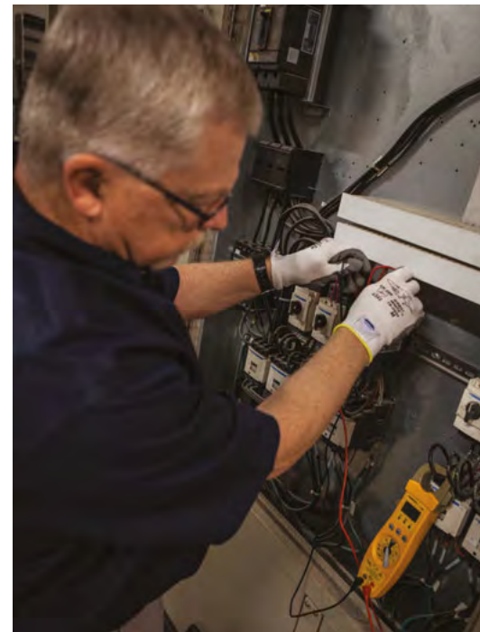
Gary Coulson, a senior HVAC technician for Brandt, uses a clamp meter to check electrical circuits. Connect from KEY2ACT lets Brandt turn data from buildings and equipment into action, pinpointing potential problems before they occur.
