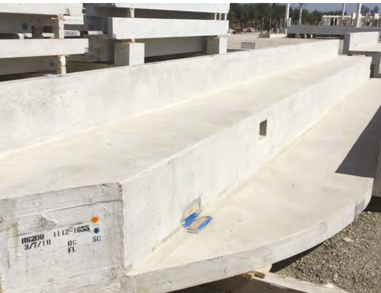
Jay R. Smith Mfg. Co. scupper drains (1520T-G-U-SSM) were integrated into the forms used to cast the concrete stadium seating sections. Smith and PPMC worked together to speed up the preparation for the precast, so that after the sections were installed, PPMC could quickly make connections and install the grate onto the drains.
