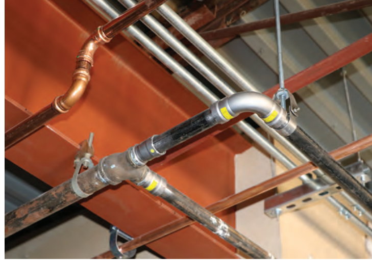
Braconier ran nearly 5,000' of new piping in the renovation and expansion of the Aims Community College welding building. It was estimated that pressing with Viega cut at least a week off the installation time in the welding lab alone.
