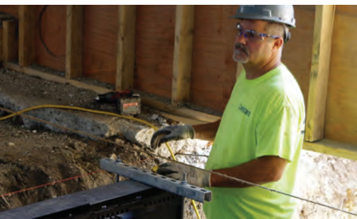
A worker begins installation of a Smith Enviro-Flo® II Trench Drain System in the facility that will be Cannistraro's manufacturing facility for plumbing, HVAC piping, fire protection, and sheet metal trades. Cannistraro was so impressed by Smith products and services that they named Smith their supplier of choice.
