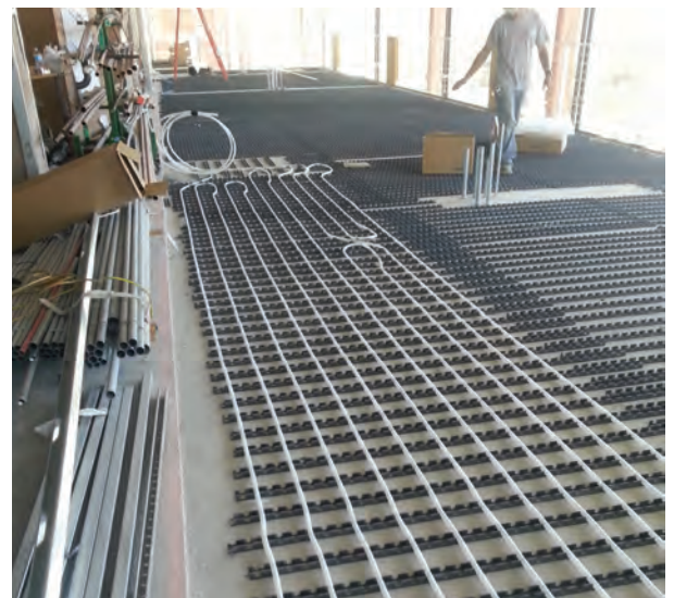
Circulating Air's four-man crew installed 16,000' of Uponor's Wirsbo hePEX tubing in UCLA's new research center. "I love how fast and easy the Uponor ProPEX system is," said Job Foreman Matt Fitzgerald.
