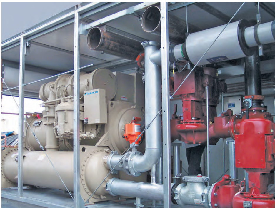
Each of the Daikin Modular Central Plants consists of a 500-ton Daikin centrifugal chiller pre-engineered with pumps, piping, cooling tower, control panel and associated water treatment system. Because they were pre-assembled, these four modules were successfully installed in just one week, resulting in no downtime for Herakles Data.
