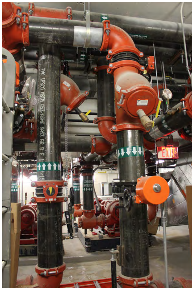
Combining Victaulic's grooved mechanical couplings with its CPS solutions significantly sped up Martin Associates' installation of an HVAC system for a new luxury apartment building in New York City. The Victaulic CPS team and Martin Associates worked closely together to fine-tune the building's piping system designs, utilizing every available inch of the tight mechanical space.
