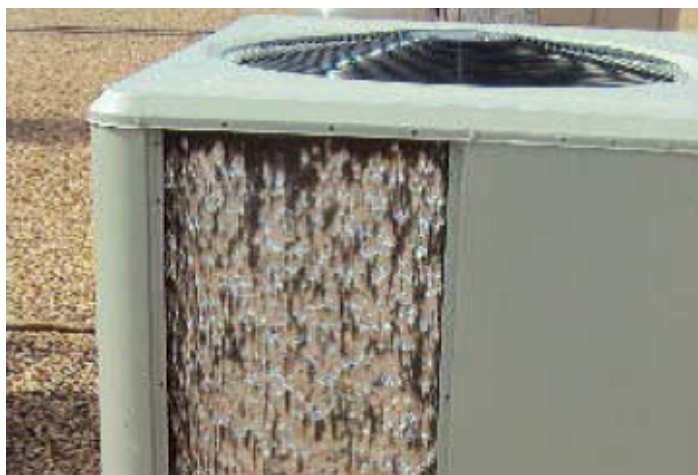
Extensive coil fin hail damage to roof and mounted HVAC unit
