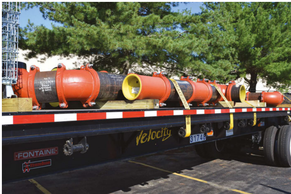
Victaulic delivered the entire mechanical room for the renovated South Street Landing Power Station to the jobsite. Overall, it took Arden less than two months to put the mechanical room together once the pieces were prepped and delivered onsite—an unachievable feat with a welded solution.
