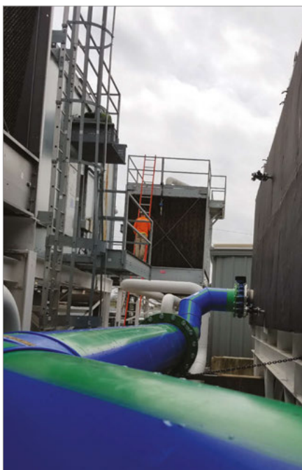
P1 Group recommended Aquatherm PP-R piping systems for Berry Global's injection-molding facility because they resist corrosion, rust, and scale, eliminating future downtime caused by pipe corrosion. Workers were able to install 300' of new pipe in just 24 hours.
