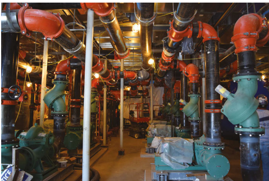
By prefabricating 90 percent of its piping and using Victaulic's grooved couplings, Arden was able to install the entire mechanical room for a massive renovation in less than two months.
