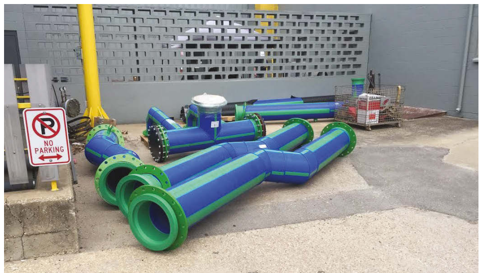
P1 Group workers quickly learned the flameless heat-fusion welding techniques required to join Aquatherm PP-R Blue Pipe, which is not only safer than traditional welding but also saves time.
