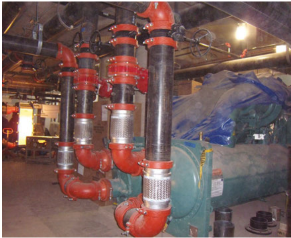
Bennell, Inc., specified Anvil's Gruvlok systems for the heating and cooling pipe of Bloomsburg University's new residence hall because they are easy to install, especially in tight spaces.
