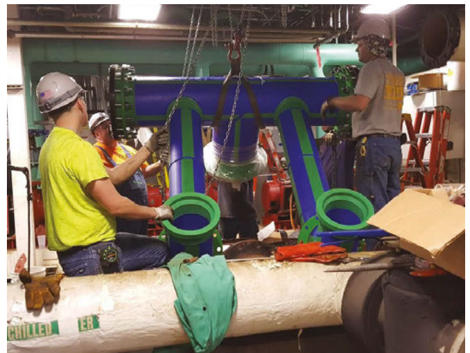
Thanks to the light weight of Aquatherm PP-R piping, P1 Group workers were able to prefabricate large sections in their shop, transport them to the jobsite, and hoist them into place quickly, saving much-needed time for a 24-hour installation job.
