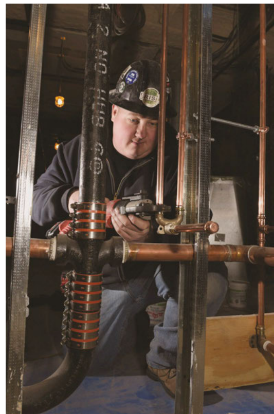
Using Viega's double drop elbow fittings allowed Commonwealth Plumbing to accommodate new sinks in the tight space of a historic building in Boston. With the pressed fittings, Commonwealth also saved time and avoided soldering.
