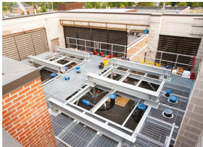
WellSpan Gettysburg Hospital’s existing cooling towers were contained by brick walls on all sides, defining the footprint. Craft & Son determined that EVAPCO towers were the only products with a small-enough footprint for the defined space yet large-enough capacity to meet the hospital’s current needs and anticipated expansion.
