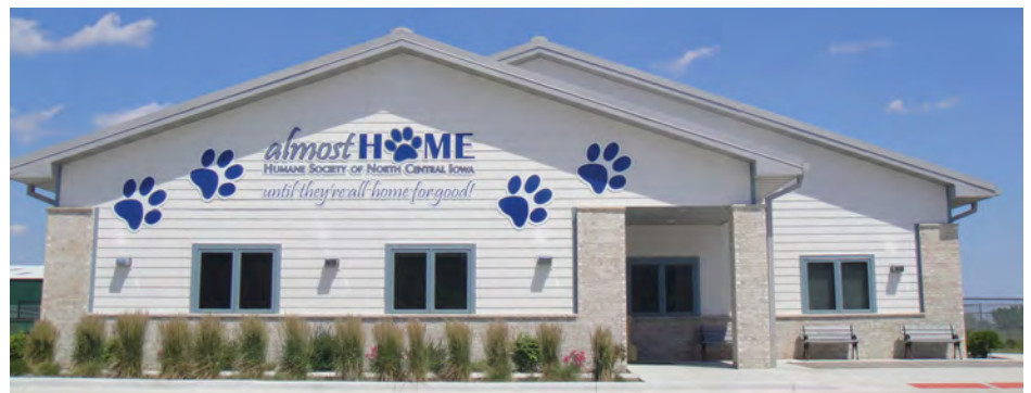
With Greenheck fans and air systems, the Almost Home Animal Shelter dramatically reduced its energy costs and improved the indoor air quality for the animals, employees, and visitors.
