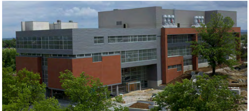
H&R Mechanical Contractors selected BAC PT2 Cooling Towers for EKU's LEED-certified, state-of-the-art science building, meeting EKU's requirements for both energy efficiency and minimal noise.
