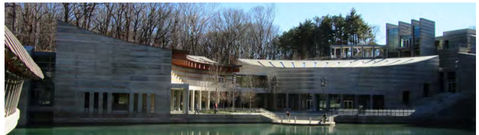
The water features of Crystal Bridge Museum posed challenges for design, construction, and installation that MMC Contractors minimized with rigorous planning and prefabrication using TSI software.
