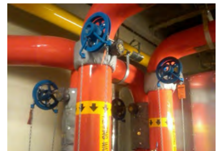
Warwick chose NIBCO's 8-inch LD-2000 lug-type butterfly valve with sprocket rim and chain because it allowed the water to flow through the bypass with no need for a special shutdown—a top priority for the hospital expansion project.
