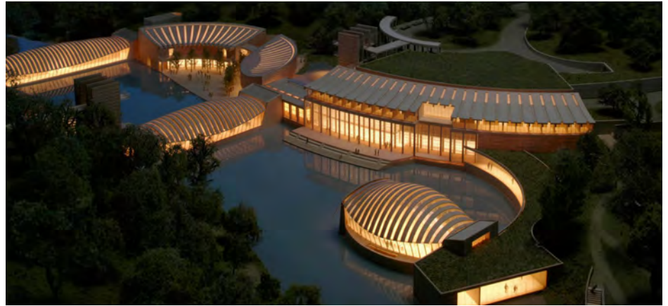
MMC Contractors relied on TSI's Autodesk and JOB-Site Solution software to model, prefabricate, and install HVAC and MEP systems for the Crystal Bridge Museum, meeting the complex demands of the design and saving time, labor, and money in the process.
