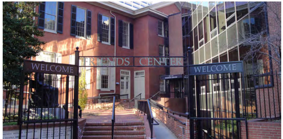
Elliot-Lewis helped the historic Friends Center in central Philadelphia upgrade its heating and cooling plant and earn LEED Platinum certification with a Carrier geothermal system, which uses the first deep (1,500 feet) wells drilled in Pennsylvania.
