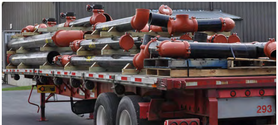
Prefabricated Victaulic pipe spools were loaded onto the truck in sequence so that they could easily be delivered to the jobsite in the right order at the right time, saving Marelich Mechanical time on the job.
