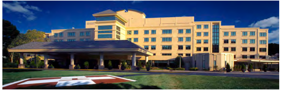
Warwick Plumbing and Heating used NIBCO products, prefabrication, and BIM to maintain uninterrupted service during construction of a new addition to the Riverside Regional Medical Center in Newport News, VA, keeping the project on track and on budget.
