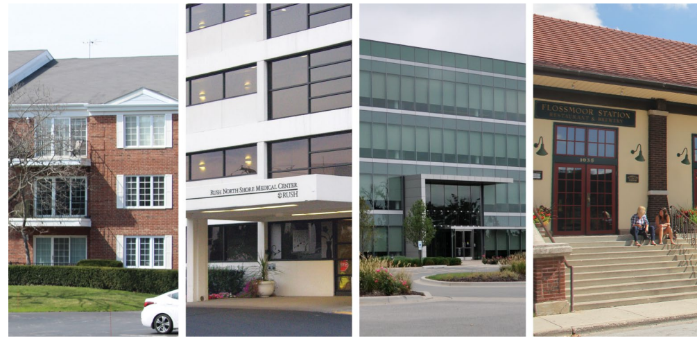
HVAC mechanical service is performed in a wide variety of buildings and facilities.
