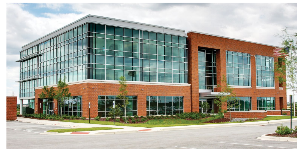
Commercial buildings with fixed glass usually require forced ventilation.
