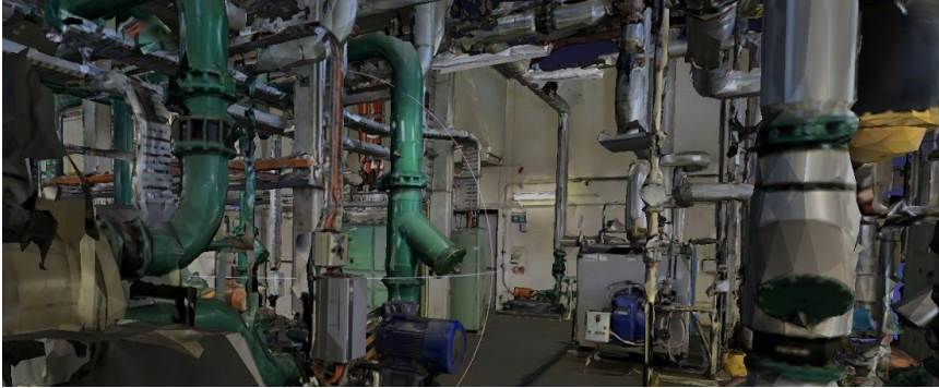
A mesh of a captured space. Notice the blocky geometry -- the angles of the real space are estimated in geometric form.
