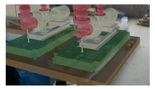
In one case, the HoloLens was brought to a project that had already installed hangers. The model was loaded for the project foreman and piping was accurately visualized running through the hangers. This made it easier to visualize the final install.
