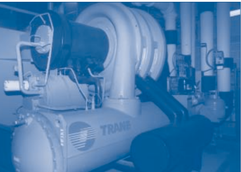
Trane Company's chillers, modular air handlers, and the Trane Tracer Summit™ building management system were selected for the Whitaker Center project.
